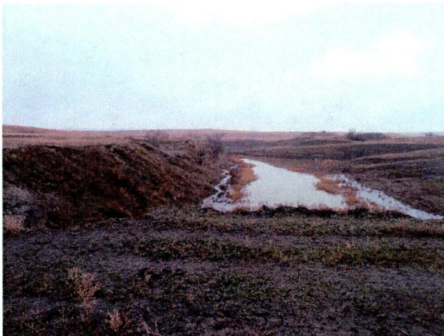
Photo 8: Photo facing east, shows highwall and pit at the Helm Brothers Site.
