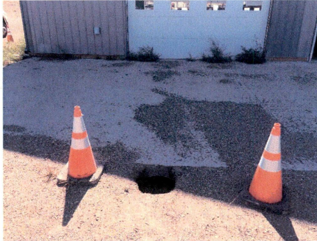
Photo 1: Williams Co Road 9 Site - Photo shows where a subsidence feature day-lighted at the edge of a concrete foundation. The sinkhole extended under the warehouse and was actively collapsing, causing structural damage to the building.
