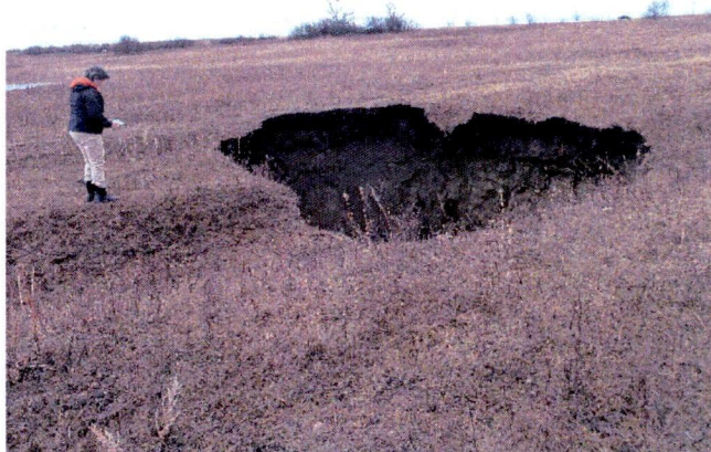
Photo 10: Photo facing west. Shows the extent of collapse at the surface. Taken 4/17/2019.
