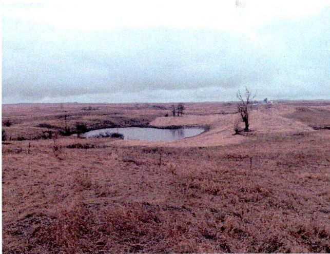
Photo 7: Post-reclamation view of the pit and former highwall at the Nilles site. Facing northwest. Shows southern pit after grading, mulching and seeding. Vegetation is starting to take hold. Taken 4/17/2019.
