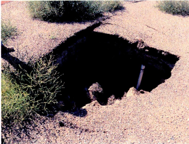
Photo 3: Williams Co Road 9 Site –This photo shows a cased borehole located immediately west of the warehouse that was swallowed by a sinkhole shortly after it was installed.
