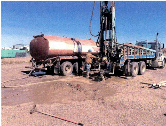
Photo 2: Williams Co Road 9 Site – Boreholes were drilled, cased and pumped with grout. This borehole was immediately north of the warehouse from Photo 1.
